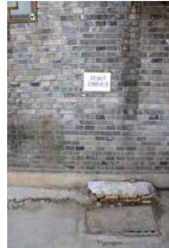
Figure 4. The covered catch basin and the warning sign on the wall (Source: author photo)
